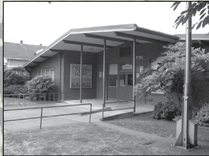
2009 photograph of main entrance
