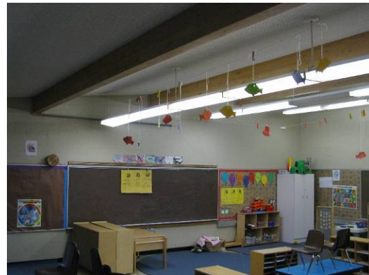
Typical classroom, note glulam roof beams (246A).
